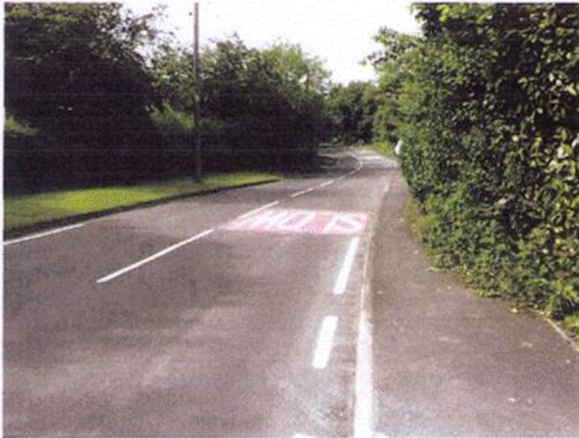
Photo 5: Visibility to right from edge of road – note front of car would be in the middle of road for driver to get this visibility.
