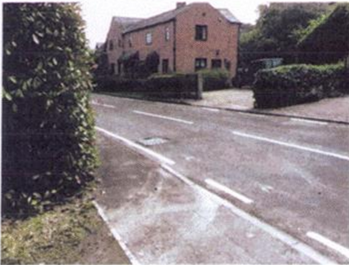
Photo 2: Visibility to the left from 2.4m in from the edge of the road at the centre of the proposed roadway.
